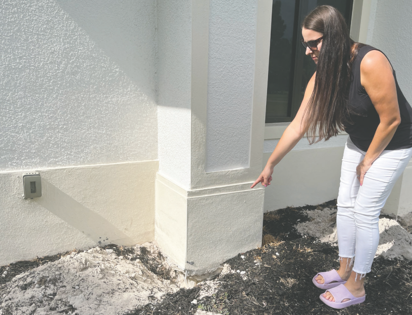
Monika Gatto can put her hand under two columns at the front of her house, where there should be footings beneath them to support the home, distribute weight and prevent settling. An X-ray scan shows there was no solid concrete footing or concrete-masonry unit block continuing below the columns. Photo by Aisling Swift
